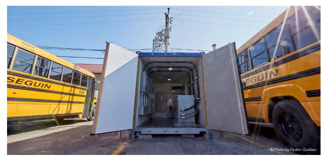
**FIGURE 5** • Installation by Cléo of a container for Autobus Séguin bus capable of supplying up to twelve 260 kW charging stations
