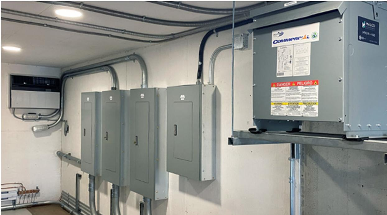
**FIGURE 11** • Autobus Maheux’s updated building electrical room to power the charging infrastructure
