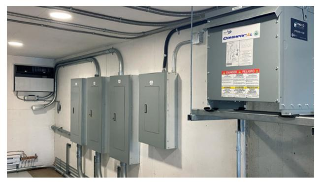
FIGURE 11 • Autobus Maheux's updated building electrical room to power the charging infrastructure
