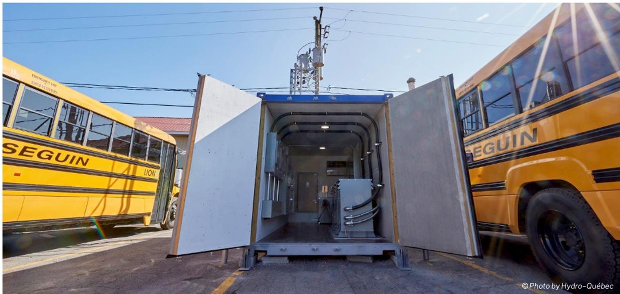
**FIGURE 5** • Installation by Cléo of a container for Autobus Séguin bus capable of supplying up to twelve 260 kW charging stations
